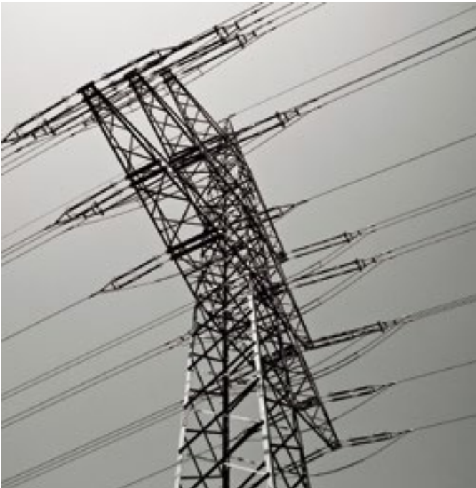
Cores of high voltage transmission lines Special alloy containing nickel and capable of withstanding temperature changes is used for this application
